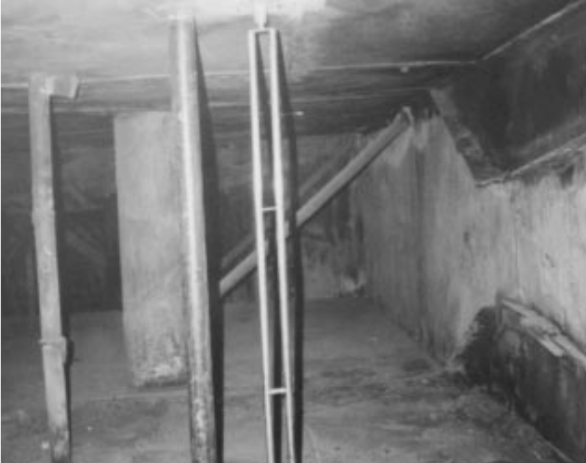
Figure 11 Secondary Air Flow Measurement
